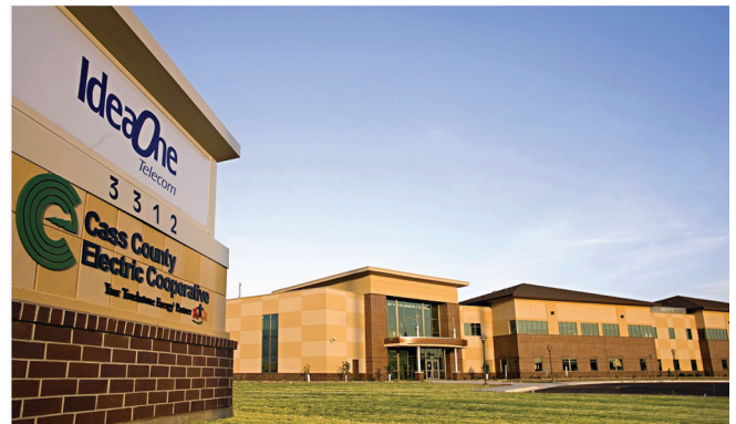
Hydromx savings resulted in ranges from 27% in August to 76% in January 2017.
